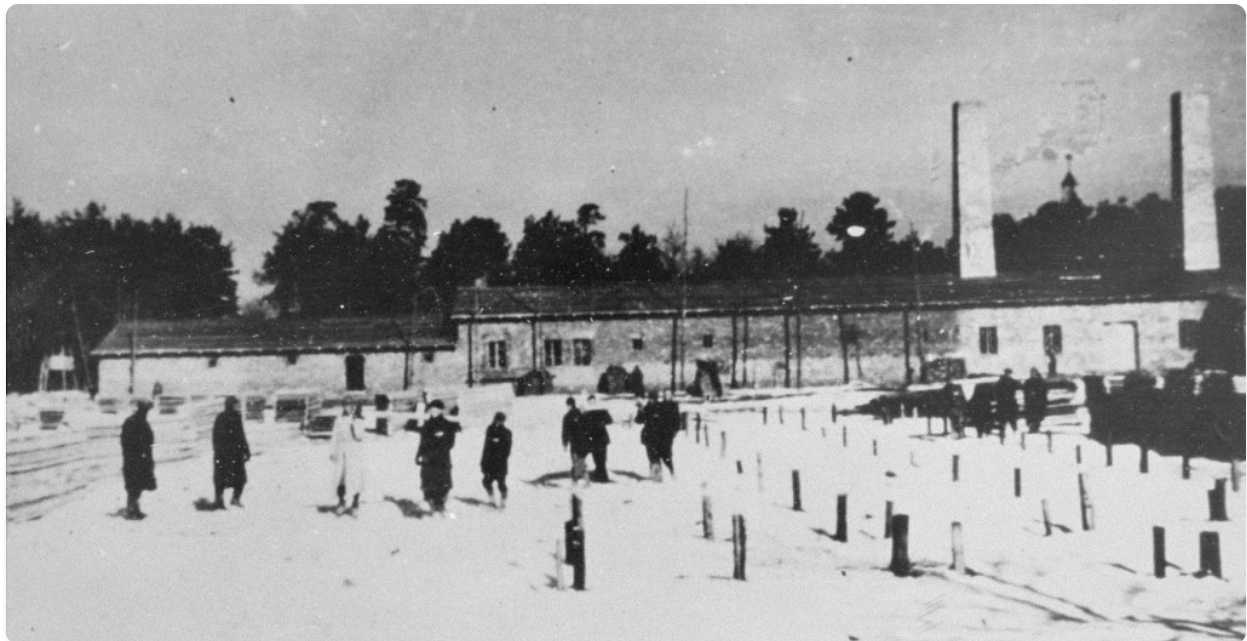
Construction of Crematorium IV at Birkenau, 1943 (built by Topf & Söhne to SS specifications). Each crematorium contained gas chambers, undressing rooms, and incineration furnaces — the apparatus the Sonderkommando were forced to operate. Most were murdered by the SS to remove witnesses.
